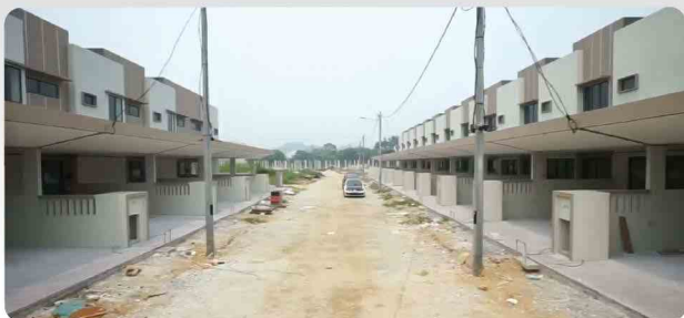
CRESCENT TERRACE CONSTRUCTION in Tanjung Malim, Perak 83 Units AirGate
