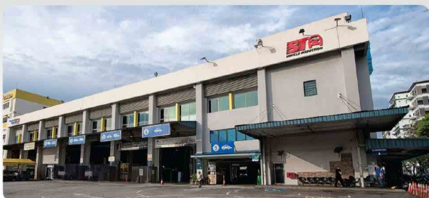
STA INSPECTION PTE LTD at Sin Ming Road, Singapore 10 Units UniGate
