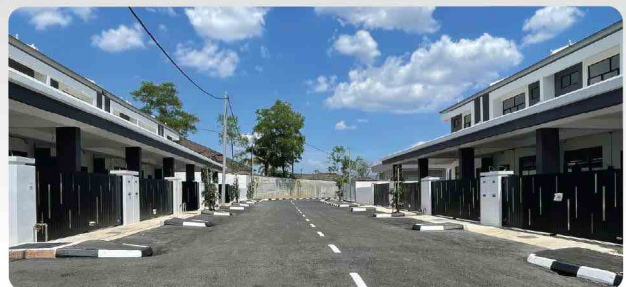
TAMAN KEMPAS in Kulim, Kedah 38 Units UniGate
